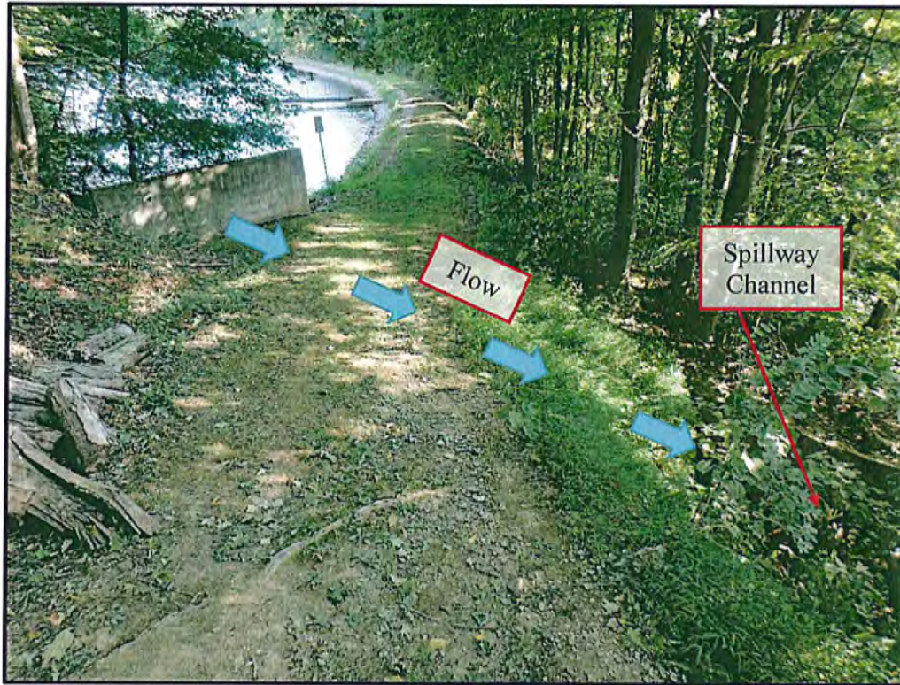
Photo 7: Principal Spillway Weir at Right Abutment – Looking Left
